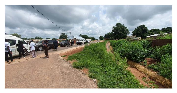
Drainage system in Upper River Region filled with sand and garbage because of soil erosion and poor waste management (sources: UNDAC)
