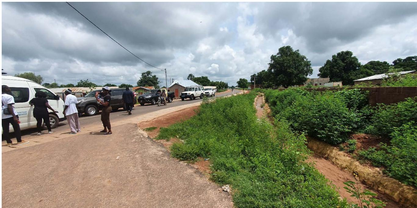
**Drainage system in Upper River Region filled with sand and garbage because of soil erosion and poor waste management (sources: UNDAC)**
